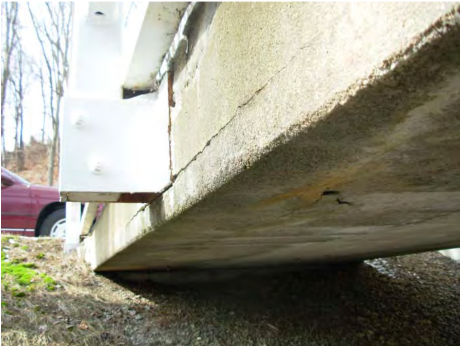
11. Bridges displaying spot cracking and spalling
