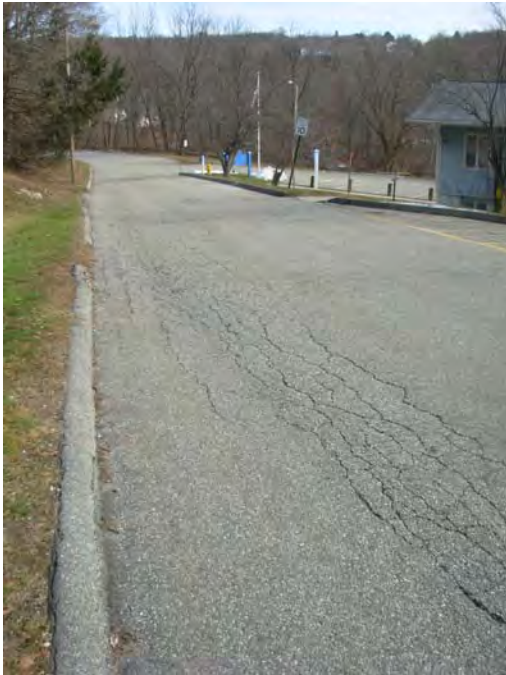
1. Cracking and settlement of access road to upper parking
