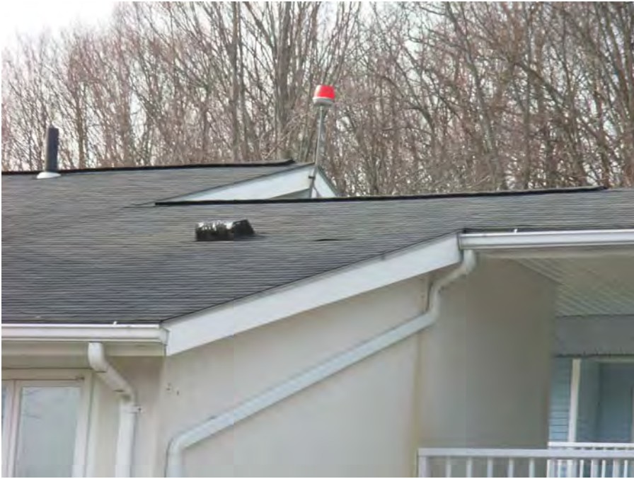
13. Spot lifting and staining of roofing shingles
