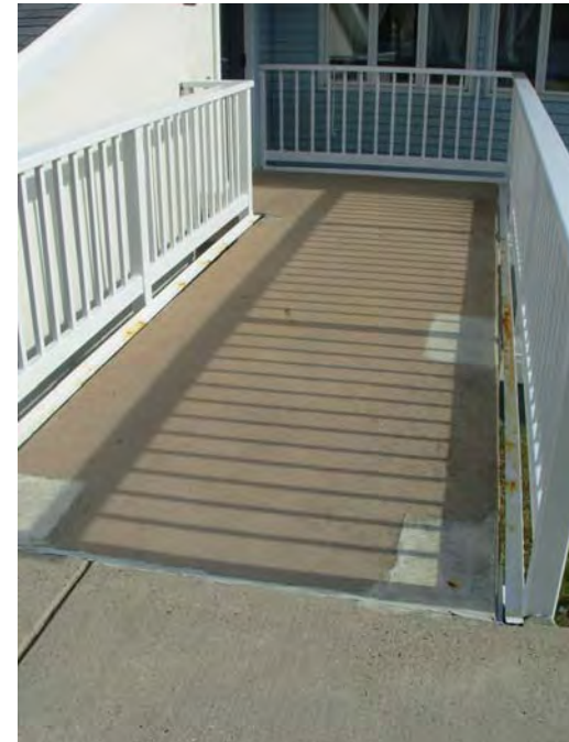
12. Patched concrete at bridges
