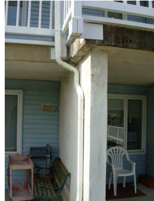
10. Spot parge coating spalling and cracking, mostly at balcony transition locations
