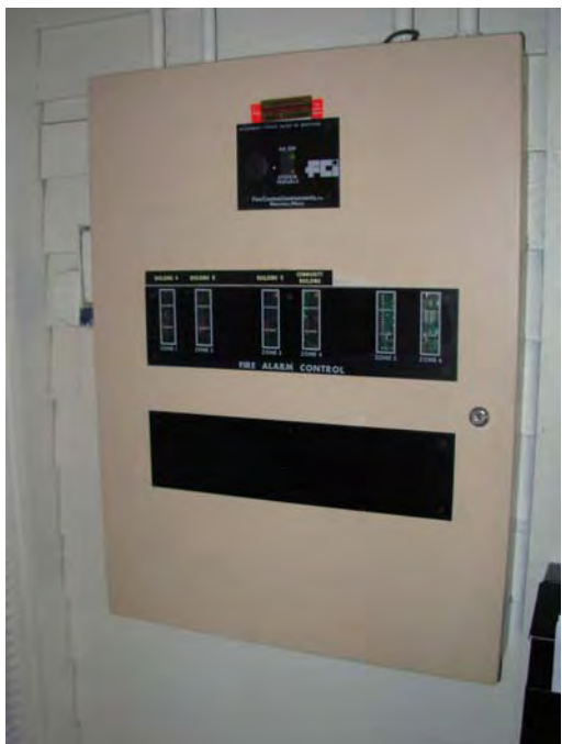
17. Fire detection - ECAS monitoring panel
