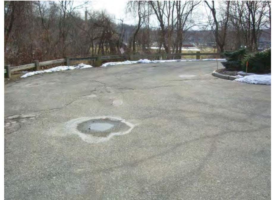
2. Cracking and settlement of lower parking area surfaces
