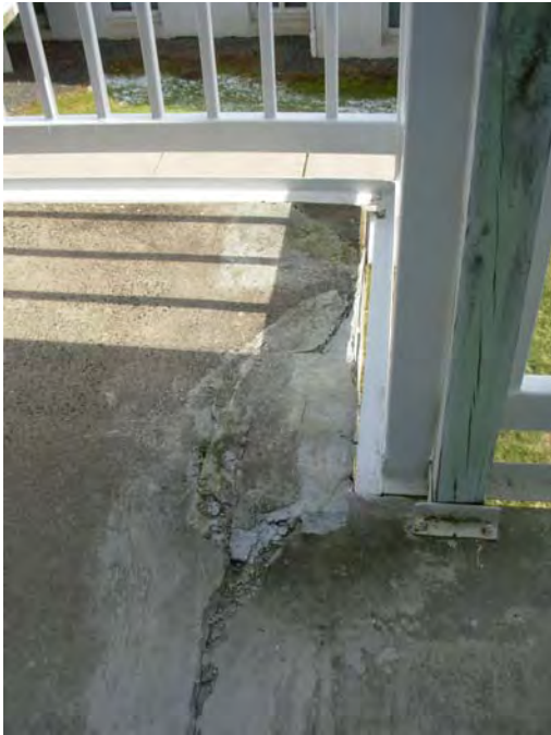
9. Spot cracking and spalling at upper balcony transitions
