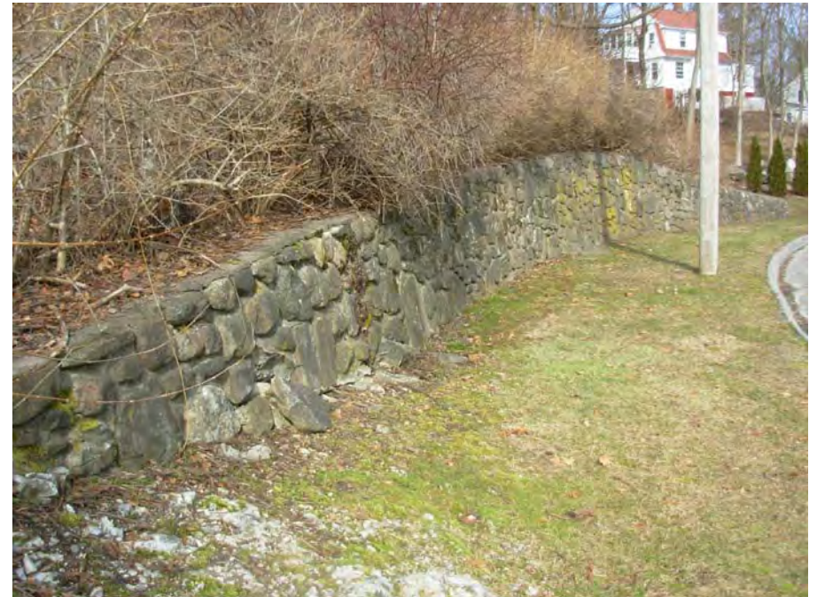
4. Some stone retaining wall deterioration
